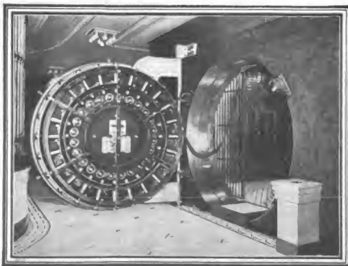
Entrance and Door to Vault.
